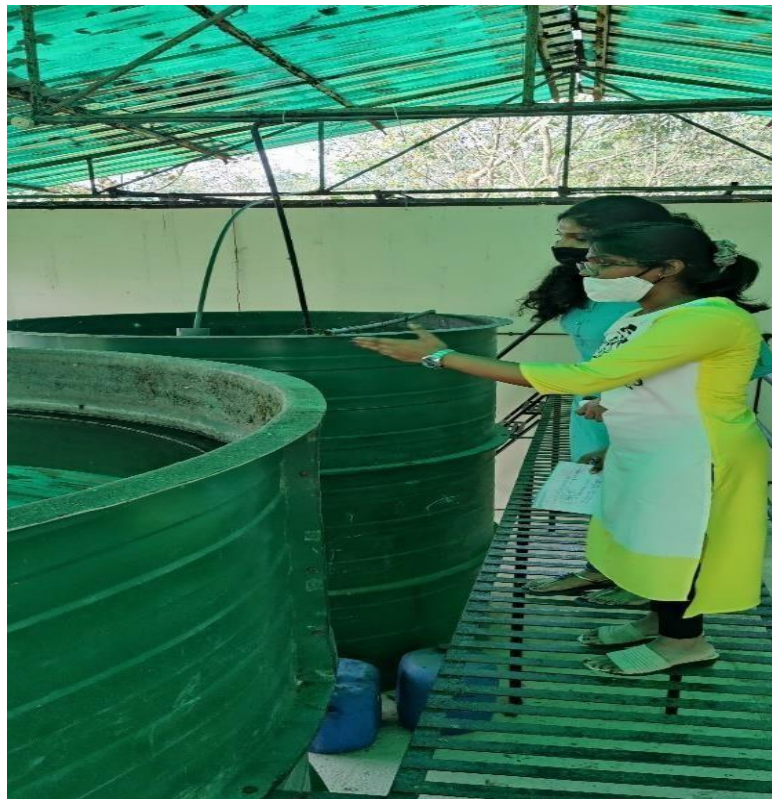
Figure 1.3 Green audit team inspecting the clarifier of ETP
