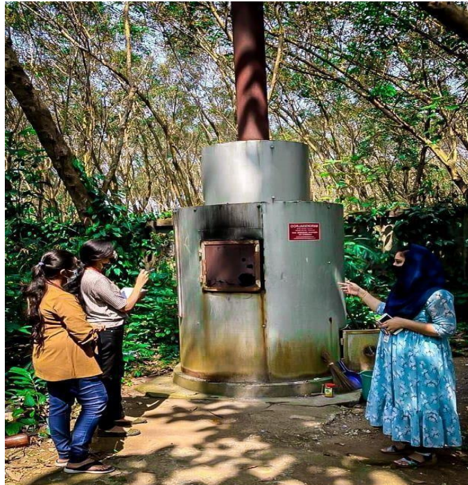
Figure 1.8 Green audit team inspecting garbage burner
